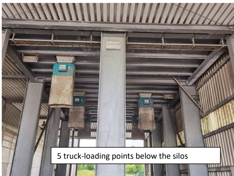
The complete steel construction is bolted and can easily be disassembled and afterwards assembled again!
