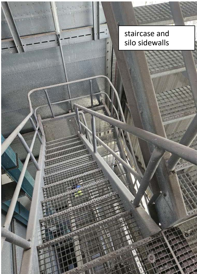
The complete steel construction is bolted and can easily be disassembled and afterwards assembled again!
