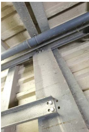
The complete steel construction is bolted and can easily be disassembled and afterwards assembled again!
